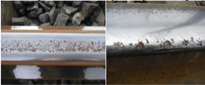
Fig. 1 Examples of worn rails (Left: Top surface worn-out, Right: Edge worn-out)
